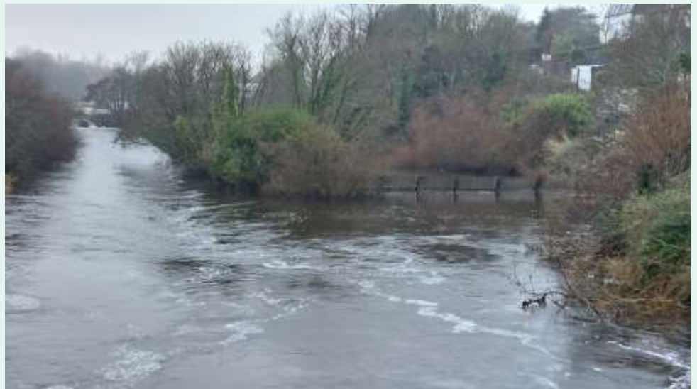
Downstream view of fence - Note high water will attract salmon towards pass. Low water conditions can lead to a buildup of adult salmon at fence
